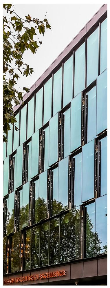
All of the Kawneer glazing systems feature a diagonal frit on the glass, with the Kawneer curtain walling featuring on the ground to top floors and the AA®100 SSG parallel-opening vents on all but the ground floor. The AA®720 doors feature on the main entrance and top floor which also features a roof terrace.
